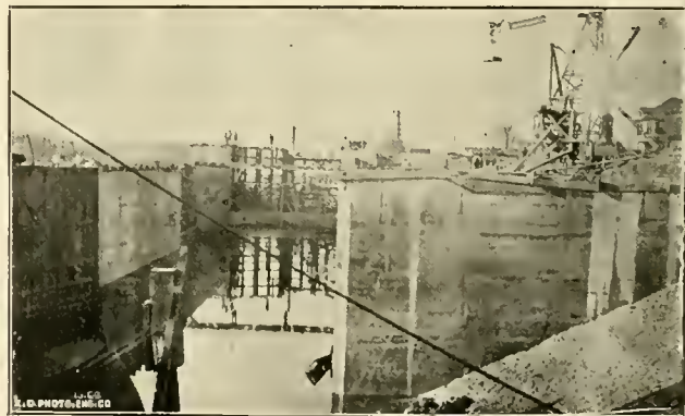
Looking Into Lock From Upper Gate, Showing Lower Gate in an Unfinished Condition.
